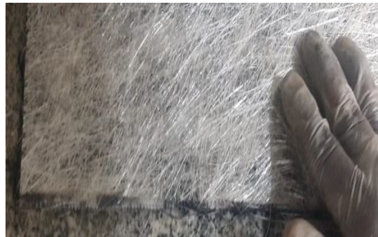
Fig 3 : Layer-02- Chopped Stranded Mat layed over layer-01
