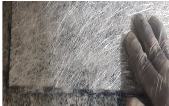
Fig 3 : Layer-02- Chopped Stranded Mat layed over layer-01
