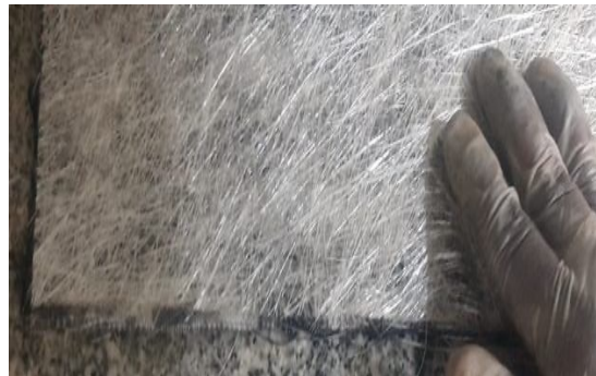
Fig 3 : Layer-02- Chopped Stranded Mat layed over layer-01
