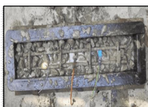
Placing the Sensors
