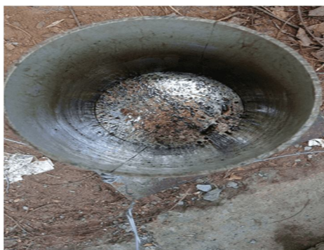
Fig 10 Greasing of Mould
