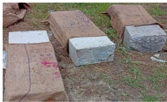
Fig 15 Curing of Beam
