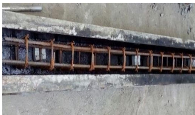
Beam Specimen with Reinforcement
