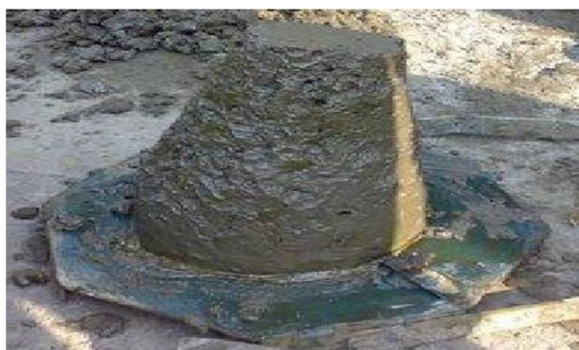
Fig. 6 - Slump cone test in progress
