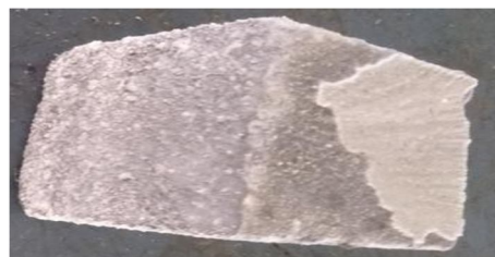
Figure 6: Sulphate Attack of Brick
