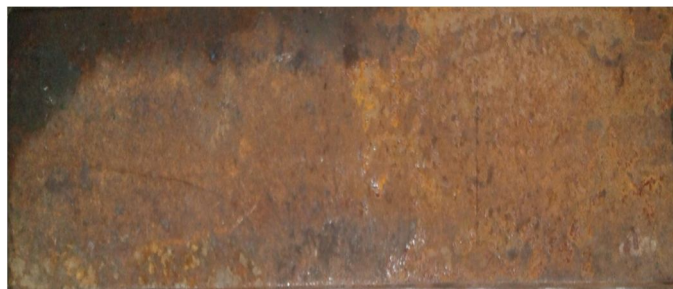
Fig. No. 4.1: Base Metal Plate before Machining.
