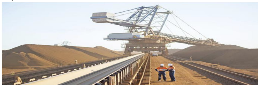
Fig. 1 The belt conveyor system (3)
