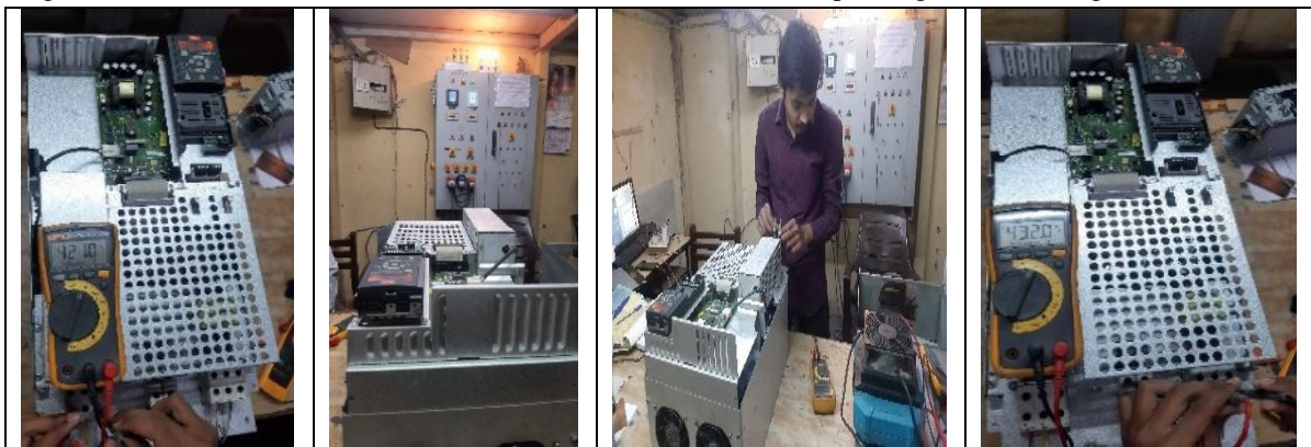
Fig.3 Hot test (power panel through) of VFD
