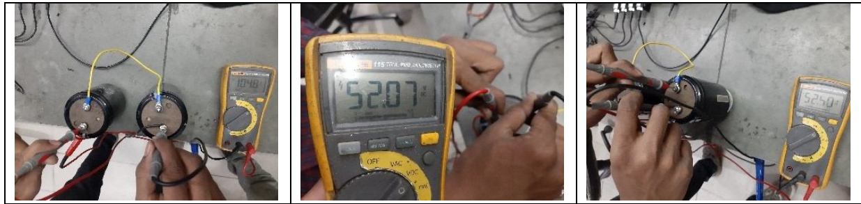
Fig.8 D.C. supply through Capacitor test
