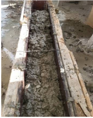
Fig. 13 Casting of Beam
