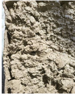
Fig. 14 Steel fibre reinforced concrete
