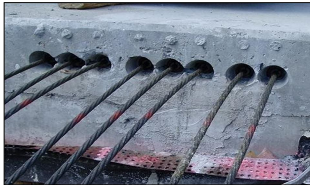
Fig.2 Tendon (cable) tails after tensioning
