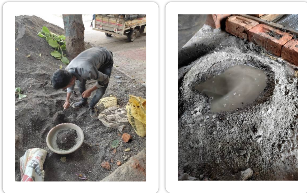
Fig. 1: Process of casting slab cube
