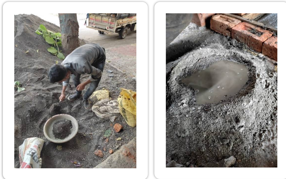
Fig. 1: Process of casting slab cube
