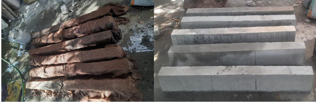
Fig. 1 Casting and Curing of Beams
