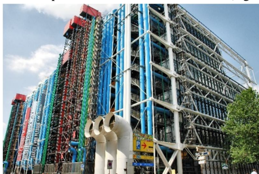
Figure 6 Pompidou Centre (Source: https://www.arrivalguides.com/en/Travelguide/PARIS/doandsee/centre-pompidou-88357 )
