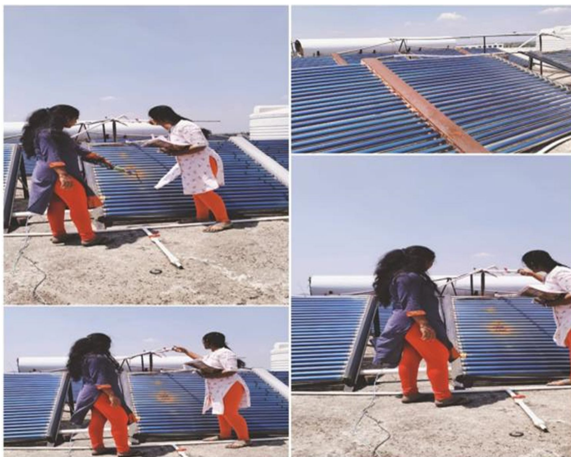
Fig6.1: Assessment of solar panel of hostel.
