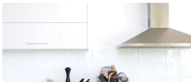
Fig No2. Ventilation at kitchen
