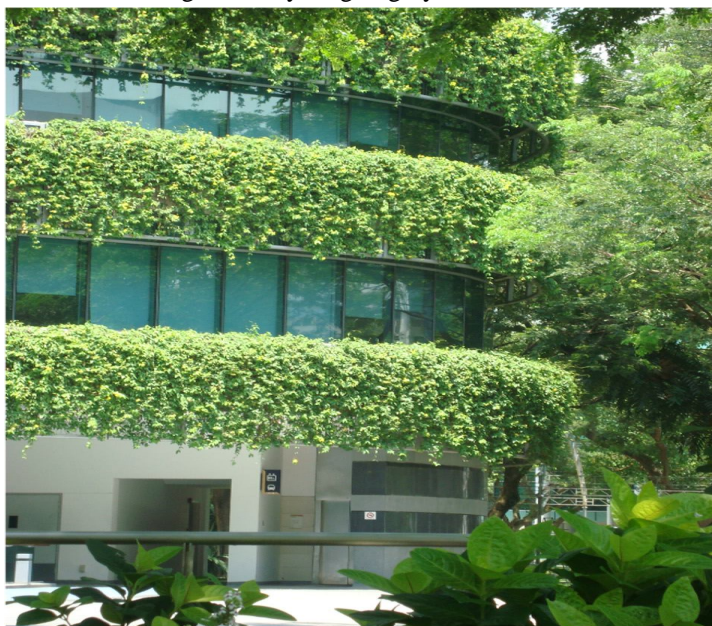
Figure 2 and 3: Greenery Integrated In Facades Has Been Successfully Applied In Buildings In Singapore And Seoul: Facade Of An Office Building In Singapore (Left) And The Internal Green Wall In The Atrium Of Seoul City Hall.
