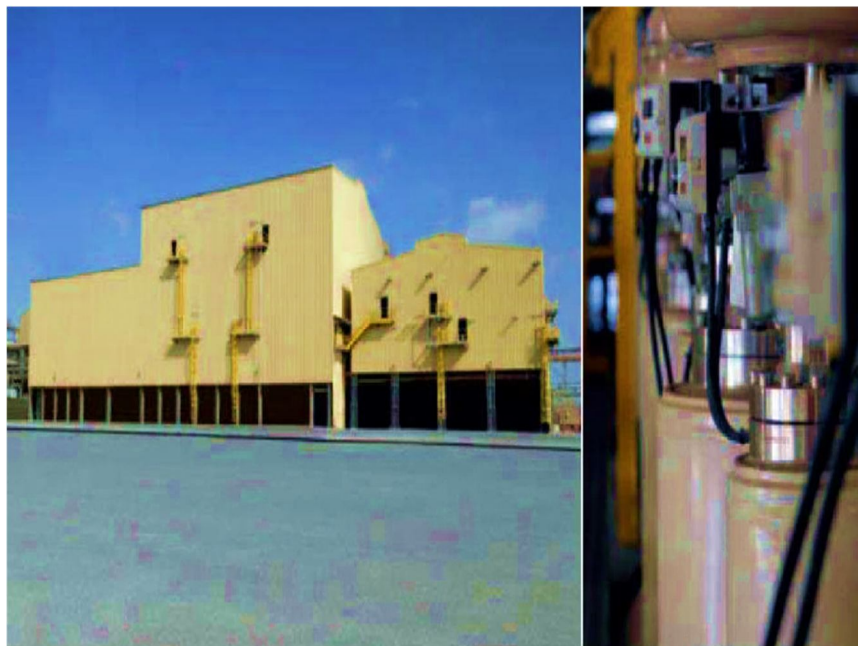
Fig 8: Conventional Helium Recovery – Helium Project of Rasgas
