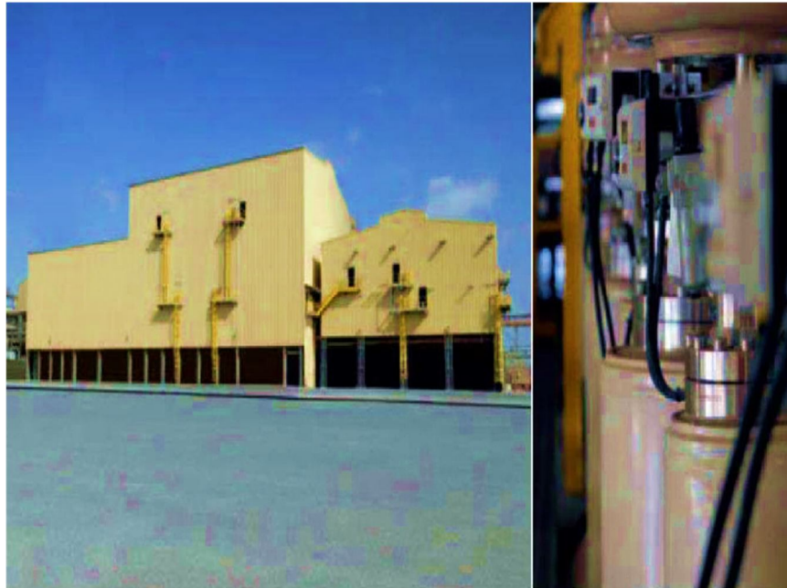
Fig 8: Conventional Helium Recovery – Helium Project of Rasgas
