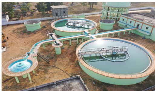
Figure-5-Clariflocculators
