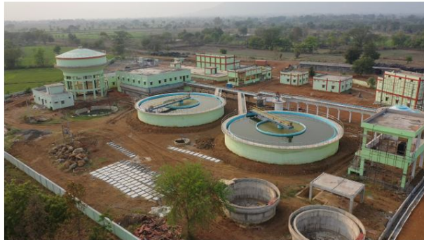
Figure-8-Construction site View
