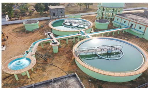
Figure-5-Clariflocculators
