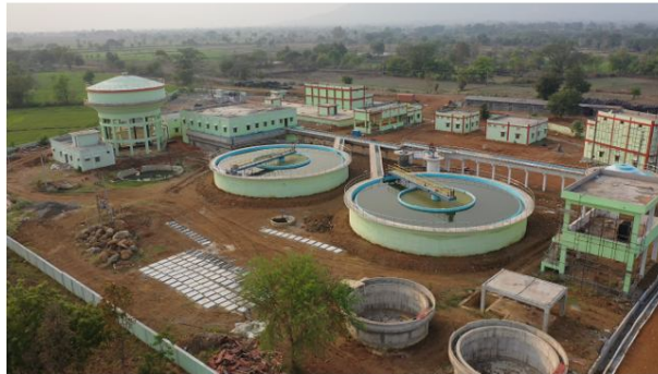
Figure-8-Construction site View
