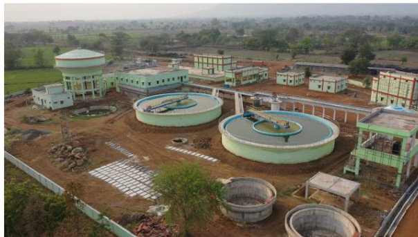
Figure-8-Construction site View
