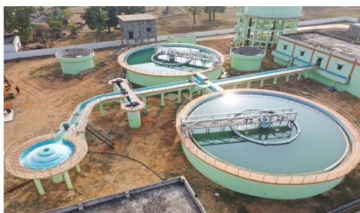
Figure-5-Clariflocculators
