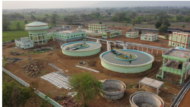
Figure-8-Construction site View
