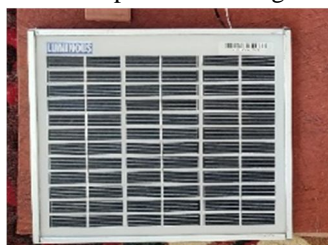
Fig. 3: Solar panel Installation
