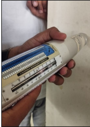
Fig. 4. Rebound Hammer Test
