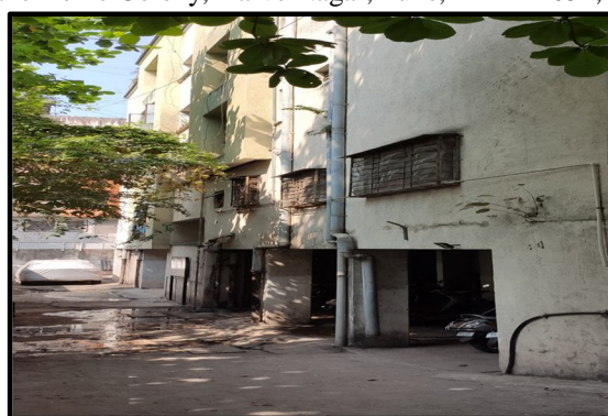
Fig. 2. Selected Building For the FMEA Process
