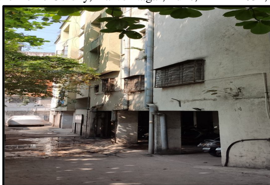
Fig. 2. Selected Building For the FMEA Process
