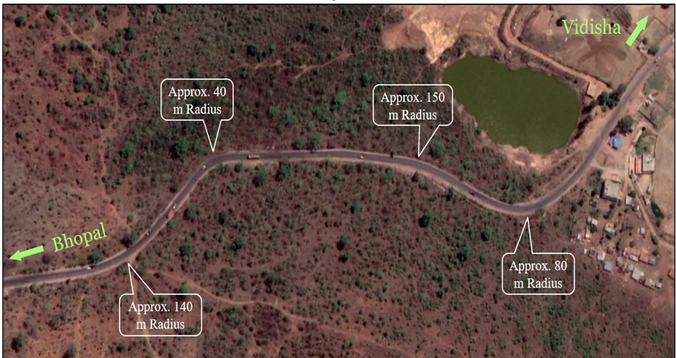
Figure 3: Horizontal curves deficiencies
