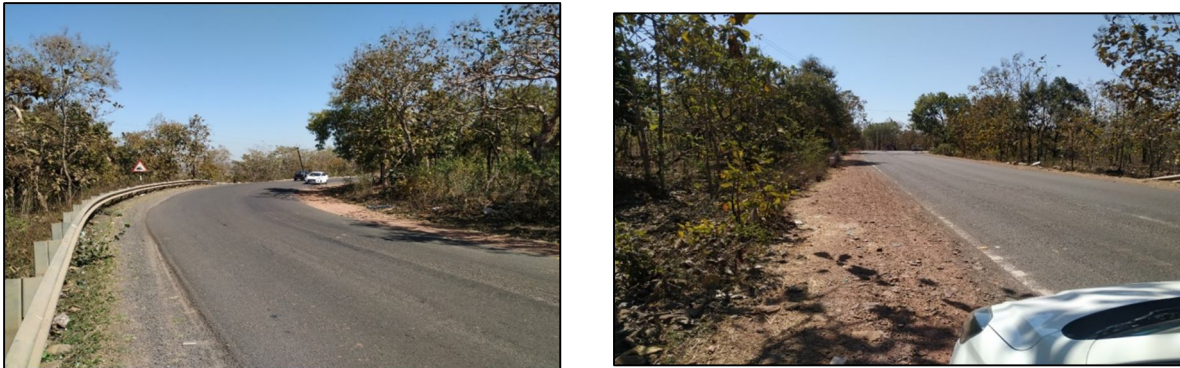
Figure 5: Balampur Ghat Section
