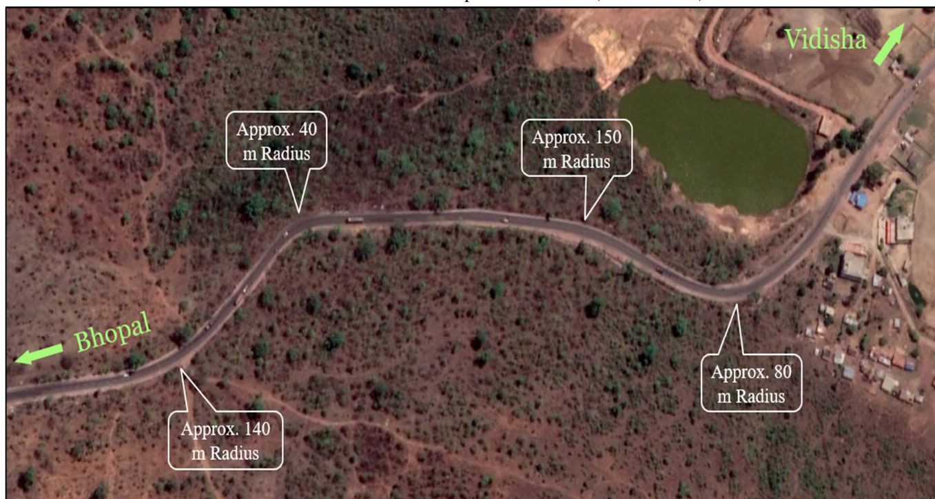
Figure 3: Horizontal curves deficiencies
