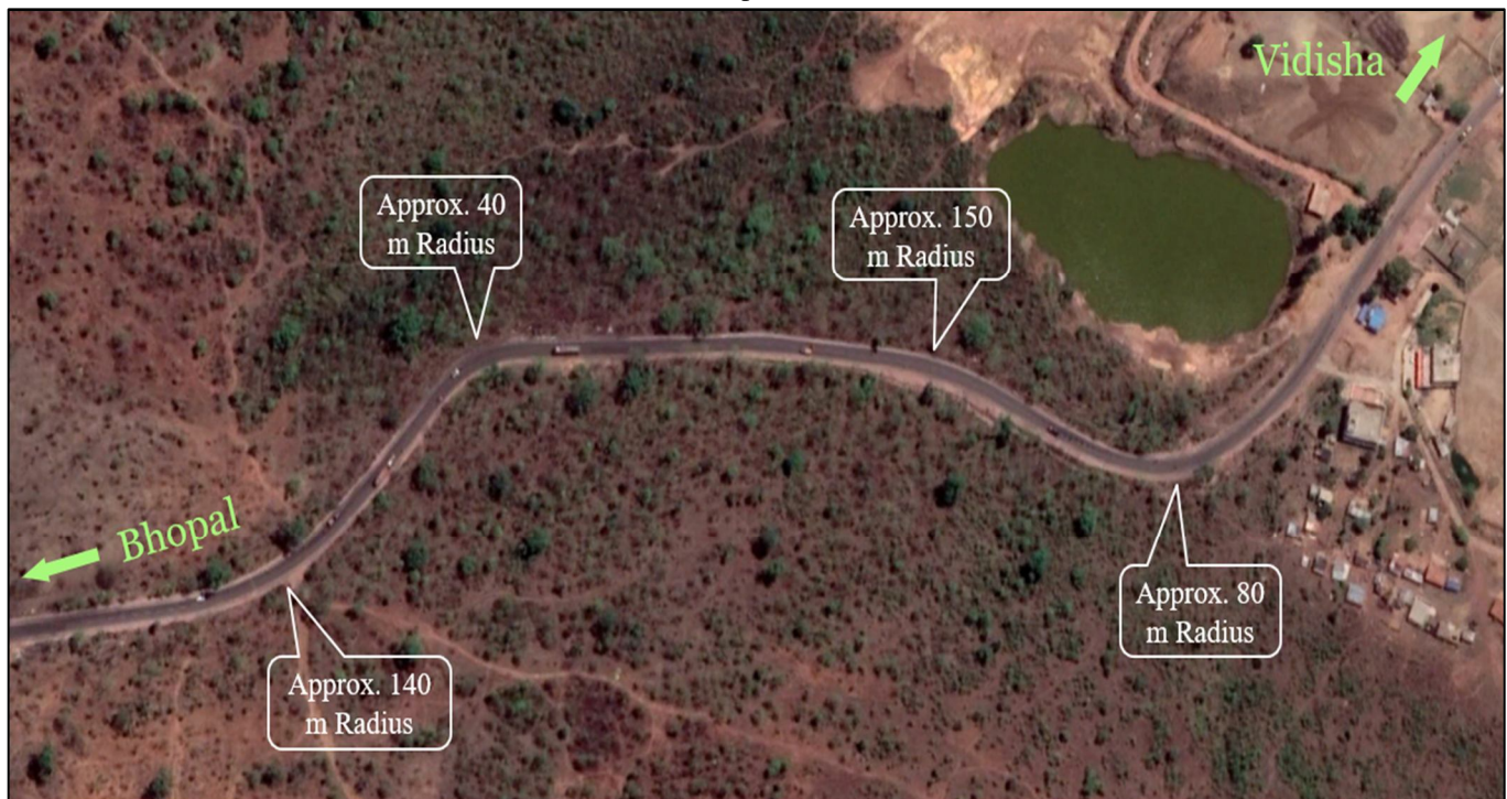
Figure 3: Horizontal curves deficiencies
