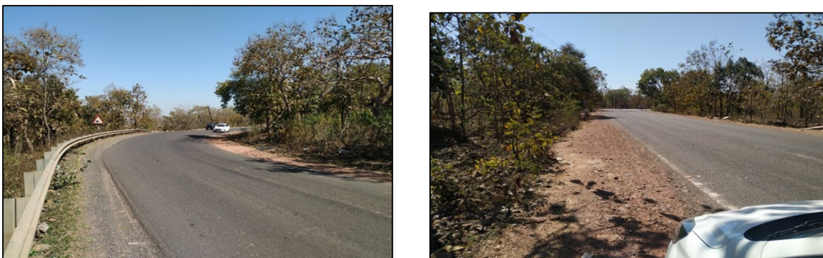
Figure 5: Balampur Ghat Section
