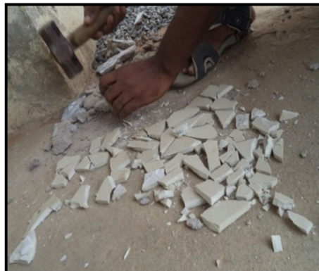
Figure 3.9: Manual Crushing Of Waste Tiles
