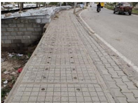
Figure 13: Good & Useable footpath Condition Source: Author
