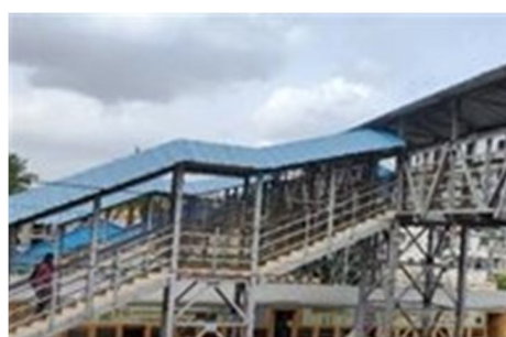
Figure 22: Foot over bridge in railway junction
