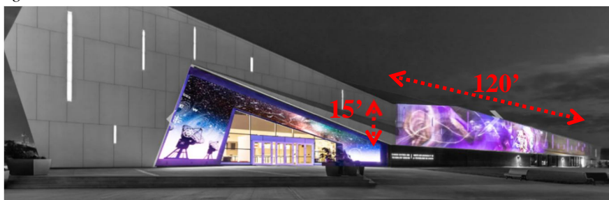
Fig. 19 – Projection Mapping on façade of Building
