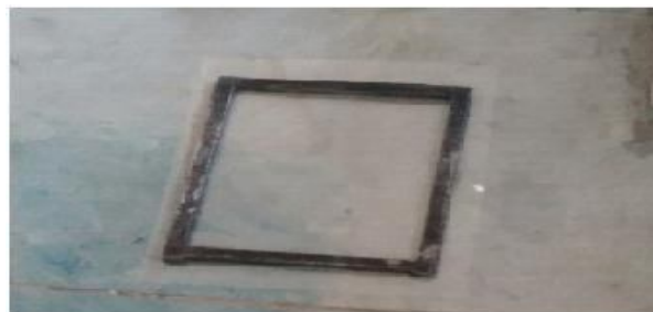
Fig3: (a) Initial setup of mould frame
