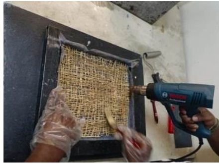
(b) During curing of the fiber plate
