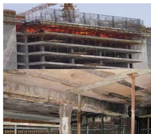
Fig no. 1 Fire Damage Beam
