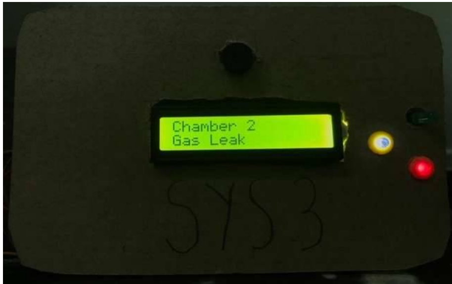
Figure 11.3 Sprinkler system during gas leak scenario
