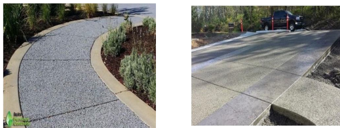
Figure 1.3: Driveways made with previous concrete
