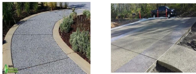
Figure 1.3: Driveways made with previous concrete
