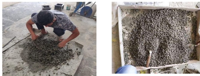
Figure 3.1 : Mixing of Pervious Concrete
