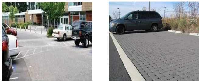
Figure 1.2 : Streets and Parking areas made with Pervious Concrete
