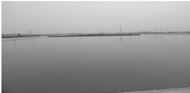
SECOND AEROBIC STABILIZATION POND, BIKANER
