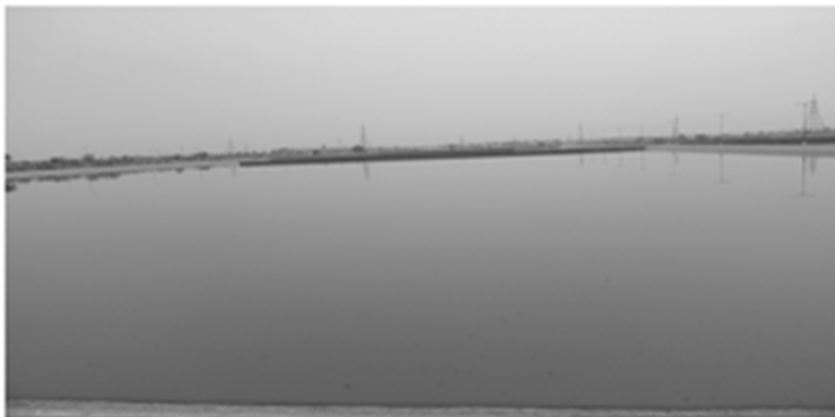
FIRST AEROBIC STABILIZATION POND, BIKANER
