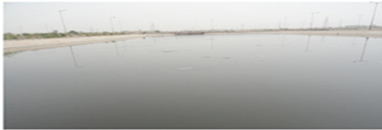
THIRD ANAEROBIC STABILIZATION POND, BIKANER PLATE : 1
