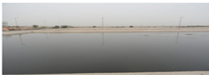
FIRST ANAEROBIC STABILIZATION POND, BIKANER
