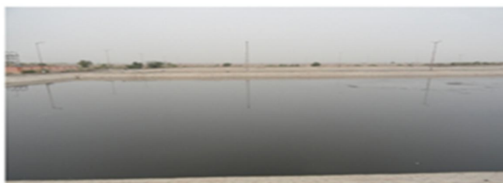
FIRST ANAEROBIC STABILIZATION POND, BIKANER
