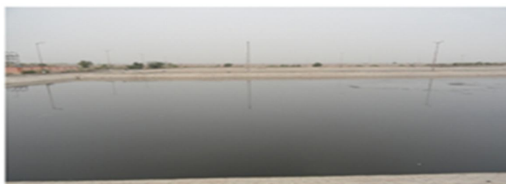
FIRST ANAEROBIC STABILIZATION POND, BIKANER
