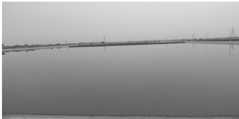
FIRST AEROBIC STABILIZATION POND, BIKANER
