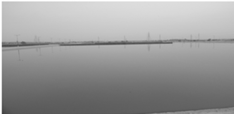
SECOND AEROBIC STABILIZATION POND, BIKANER
