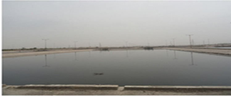
SECOND ANAEROBIC STABILIZATION POND, BIKANER
