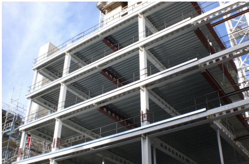
Figure E.3 Composite Construction
