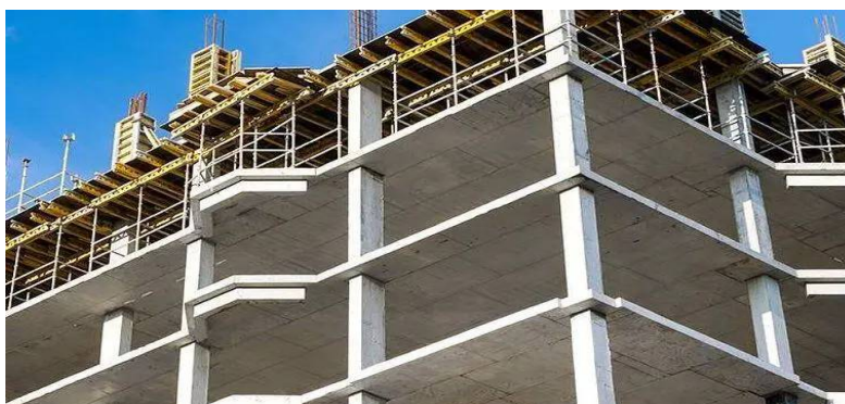
Figure E.2 Reinforced Concrete Construction
