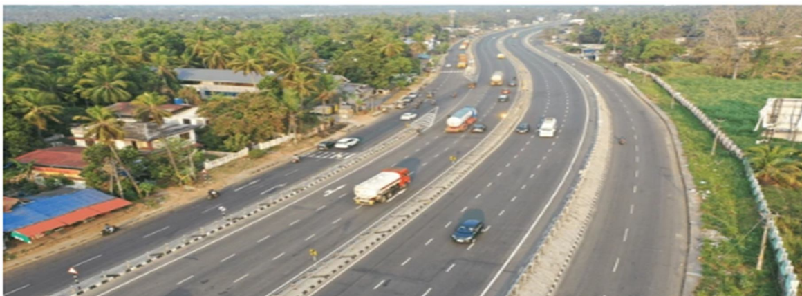
Fig 2: New Six Lane National Highway (NH-66) in Kerala
