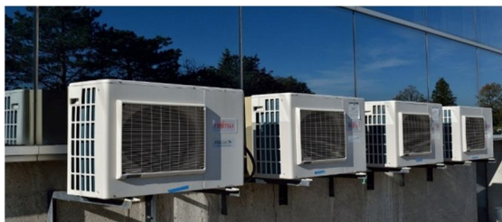
Fig a) An array of air conditioner condenser units outside a commercial office building
