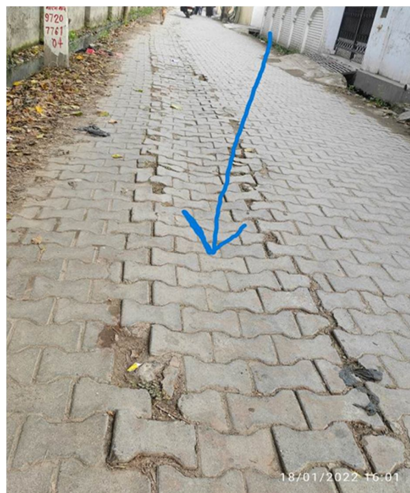
Figure 7 Interlocking Bricks Roads Settlement
