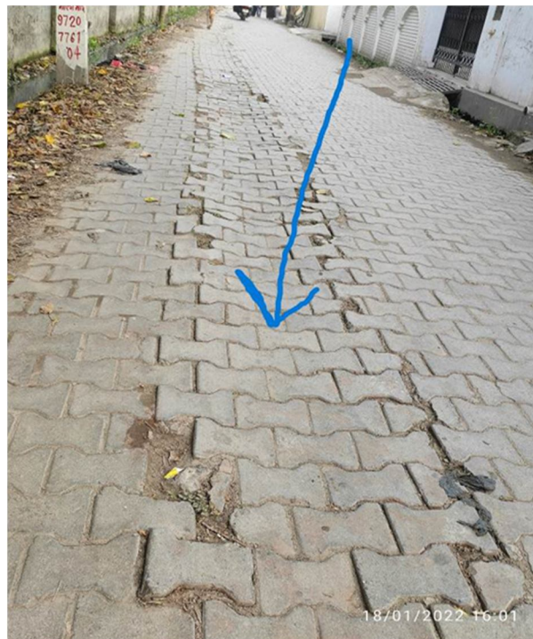
Figure 7 Interlocking Bricks Roads Settlement
