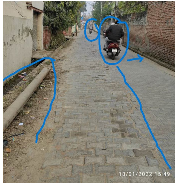
Figure 20 Pole and users moving on wrong hand
