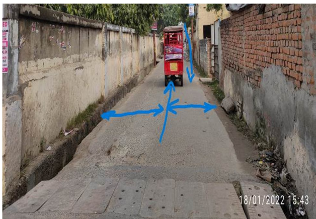
Figure 15 Less path for moving vehicles and moving on wrong hand
