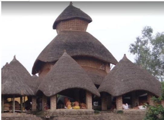
Figure 10- gurukul uses vernacular architecture of Bengal.
