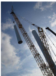
Figure.2.Erection of Tower cells & Blades
