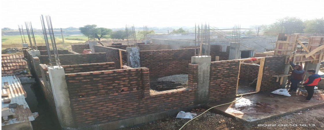
Site for casting mould
