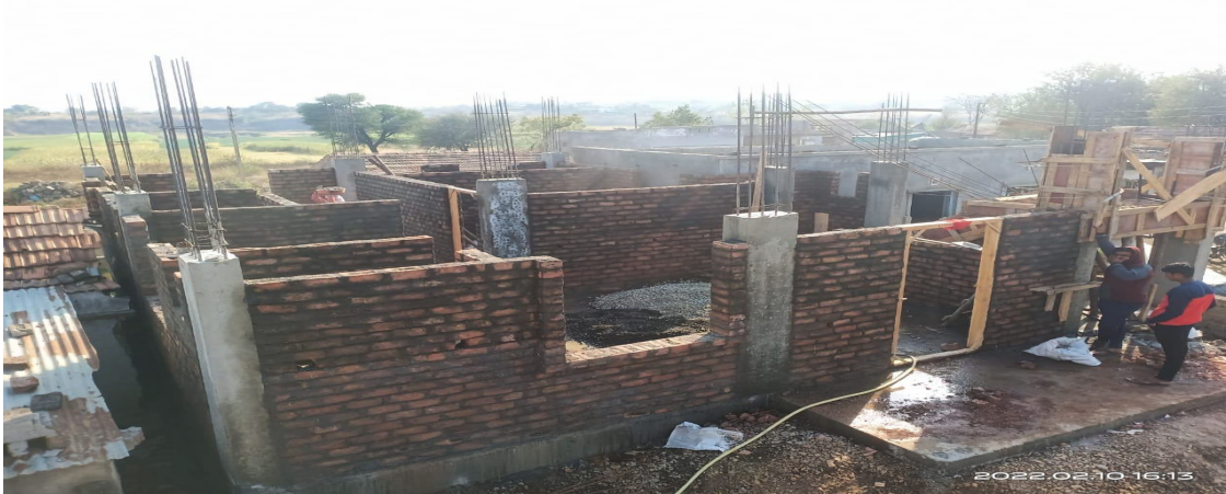
Site for casting mould
