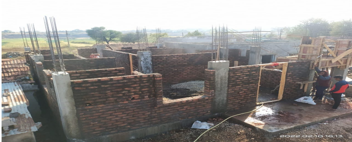
Site for casting mould
