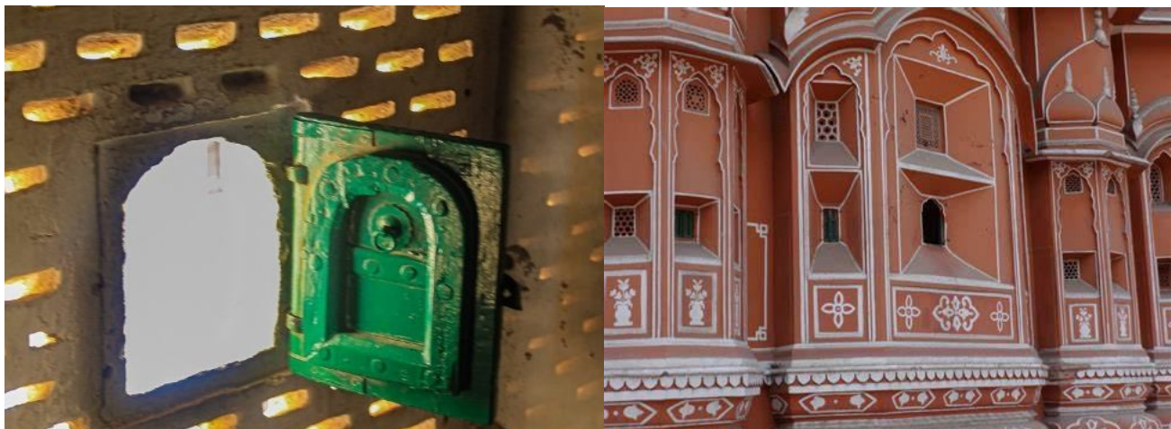
Figure 12: Small windows and cut outs in the facade of Hawa Mahal
