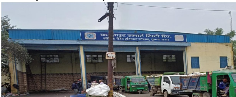
Fig-2: Transfer Station of zone 2
