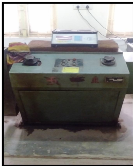
Figure 5: Hydraulic system control
