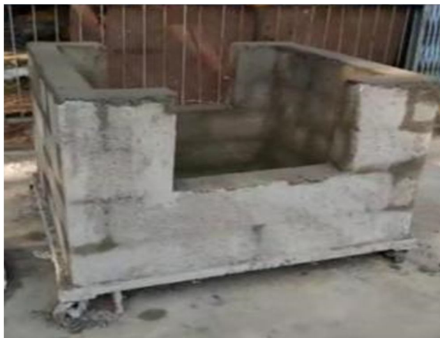
Fig. 2 The room ready with plastering
