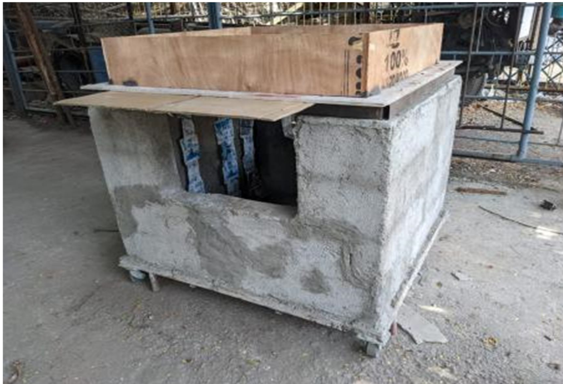
Fig. 7 Prototype room with all passive cooling techniques
