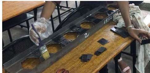
Fig. 9 Applying adhesive on castellated beam
