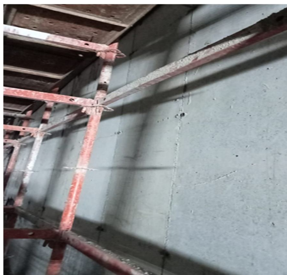
Fig 13. Smooth surfaces of the cast in situ high performance flowable concrete
