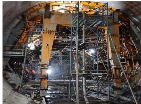
Fig 12 Actual site photographs during concrete placing at site showing two stages of concrete pouring and nos of bends to reach at placement point.
