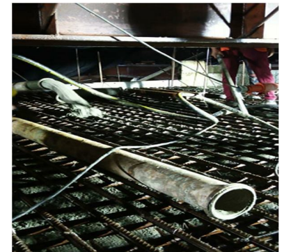
Fig 12 Actual site photographs during concrete placing at site showing two stages of concrete pouring and nos of bends to reach at placement point.
