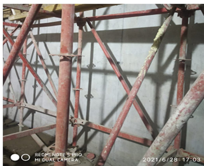
Fig 13. Smooth surfaces of the cast in situ high performance flowable concrete
