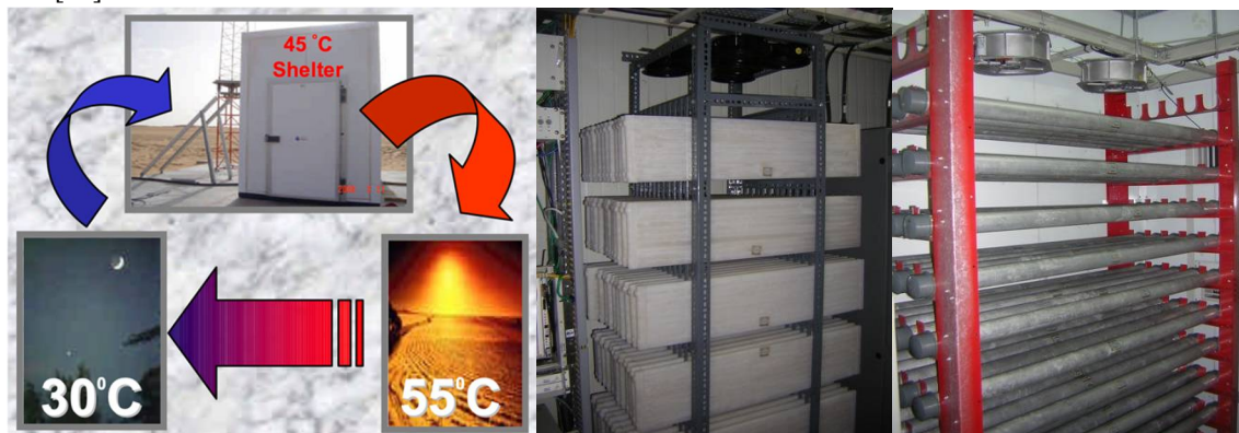
Fig 11. Thermal management in telecom shelters using HDPE panels and aluminum pipes filled with PCM and stacked neatly.
