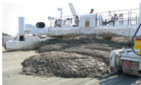
Fig. 1. Concrete mixing plant
