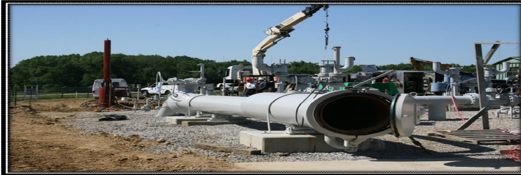
Figure 2. Pigging Pipeline
