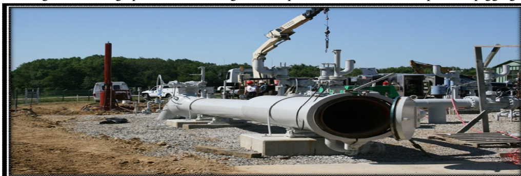
Figure 2. Pigging Pipeline
