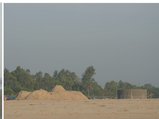
Tajpur Watch Tower Construction, 2020
