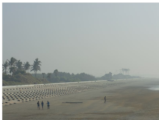
Digha Marine Drive construction, 2020
