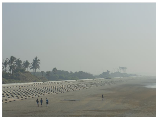
Digha Marine Drive construction, 2020
