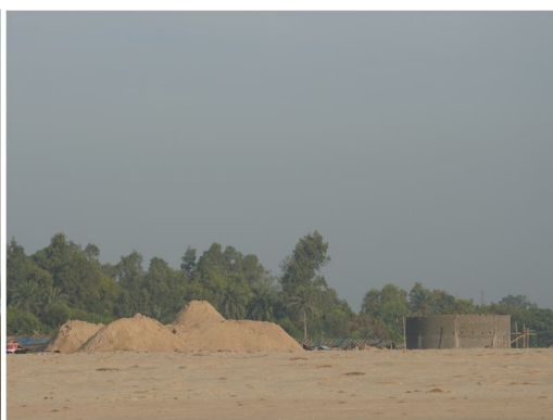
Tajpur Watch Tower Construction, 2020
