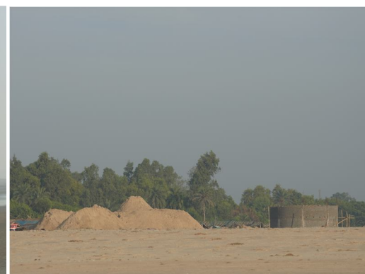
Tajpur Watch Tower Construction, 2020
