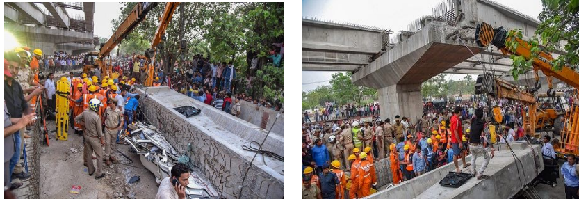
Fig 1.2:- Varanasi UP Flyover Girders collapse on 15-May-2018
