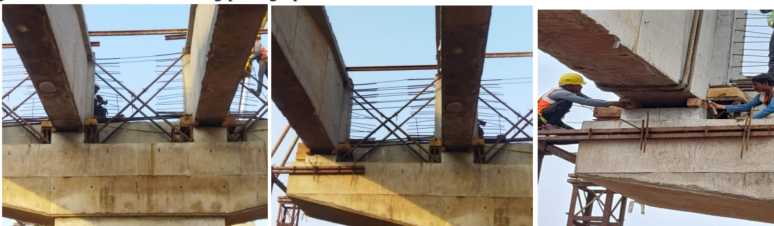
Fig 1.3:- Supporting arrangement of PSC Girdes (3 Photos)
