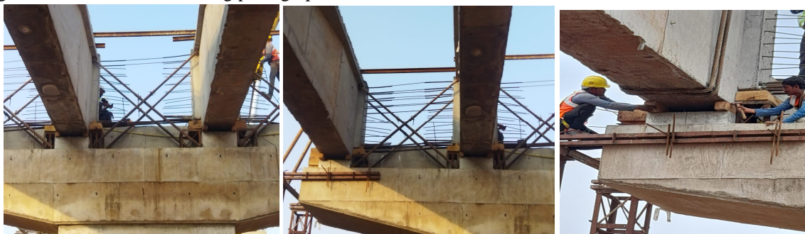
Fig 1.3:- Supporting arrangement of PSC Girdes (3 Photos)
