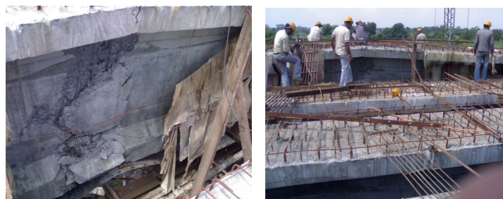
Fig 3.1:- Crushing of concrete at weak flexural zone due to insufficient conc strength
