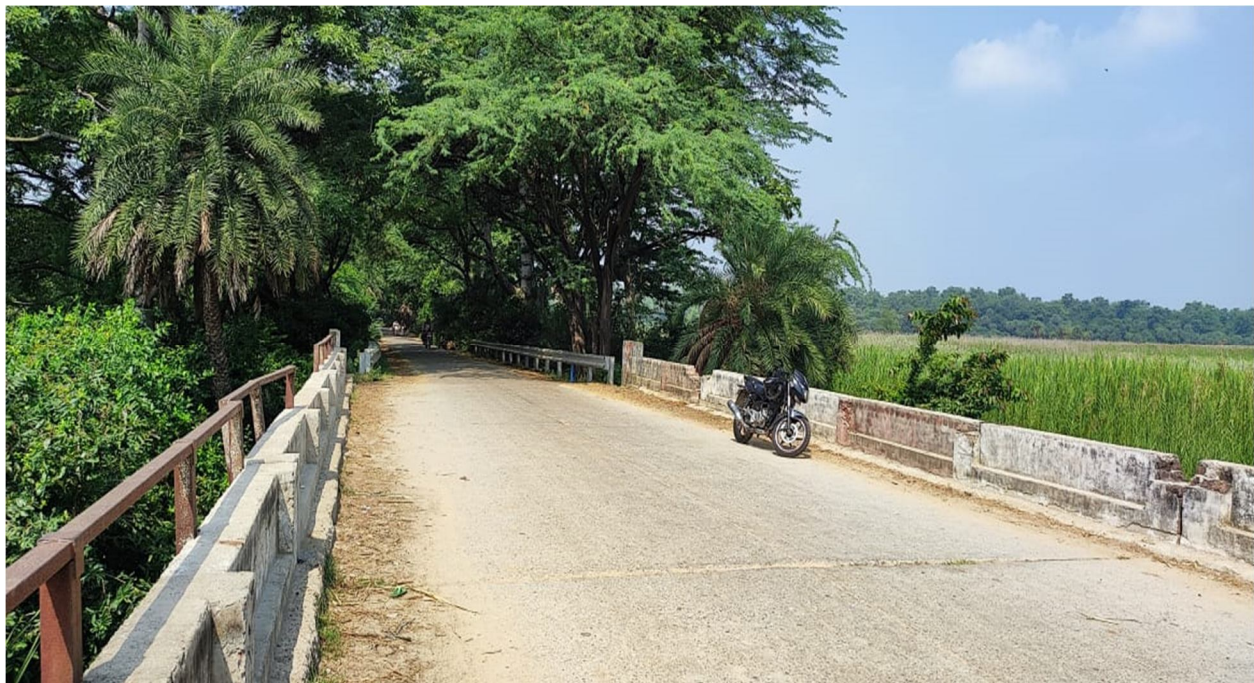
Image 14: Bridge on Budhi Ganga at Dayalpur (Tehsil Mawana, District Meerut)
