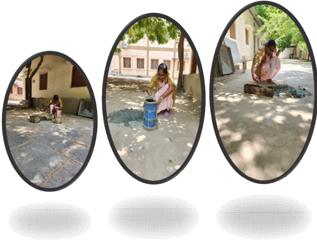
Fig 4. Casting of Moulds
